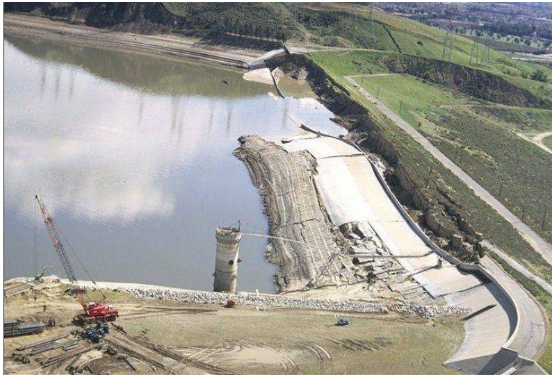
Figure 1.4 - Diffuse rupture of San Fernando dam, United States 1971
