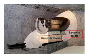
Figure 1. Nagra concept, based on bentonite blocks and bentonite pellets.
