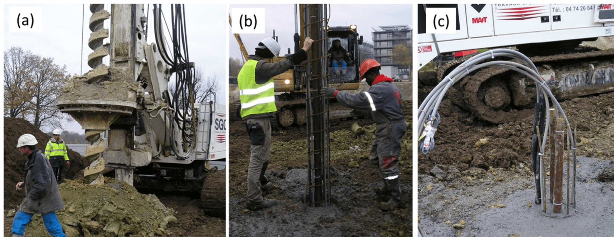
Fig. 3.8 Pile installation by Continuous Flight Auger (CFA) method: drilling & concrete casting (a); installing the reinforcement cage (b); work completed (c).
