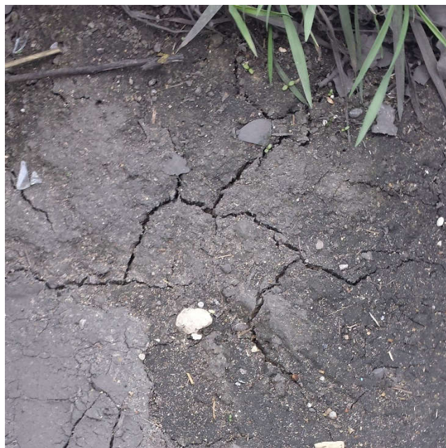
Figure 68 : Cracks in the BFS filter media in February 2017
