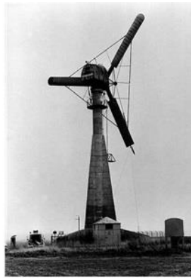
1957: Johannes Juul, Gedser, Denmark 3-bladed, pitch-controlled HAWT
