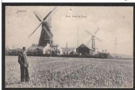
1891: Poul la Cour, Askov, Denmark first big-scale HAWT test rig
