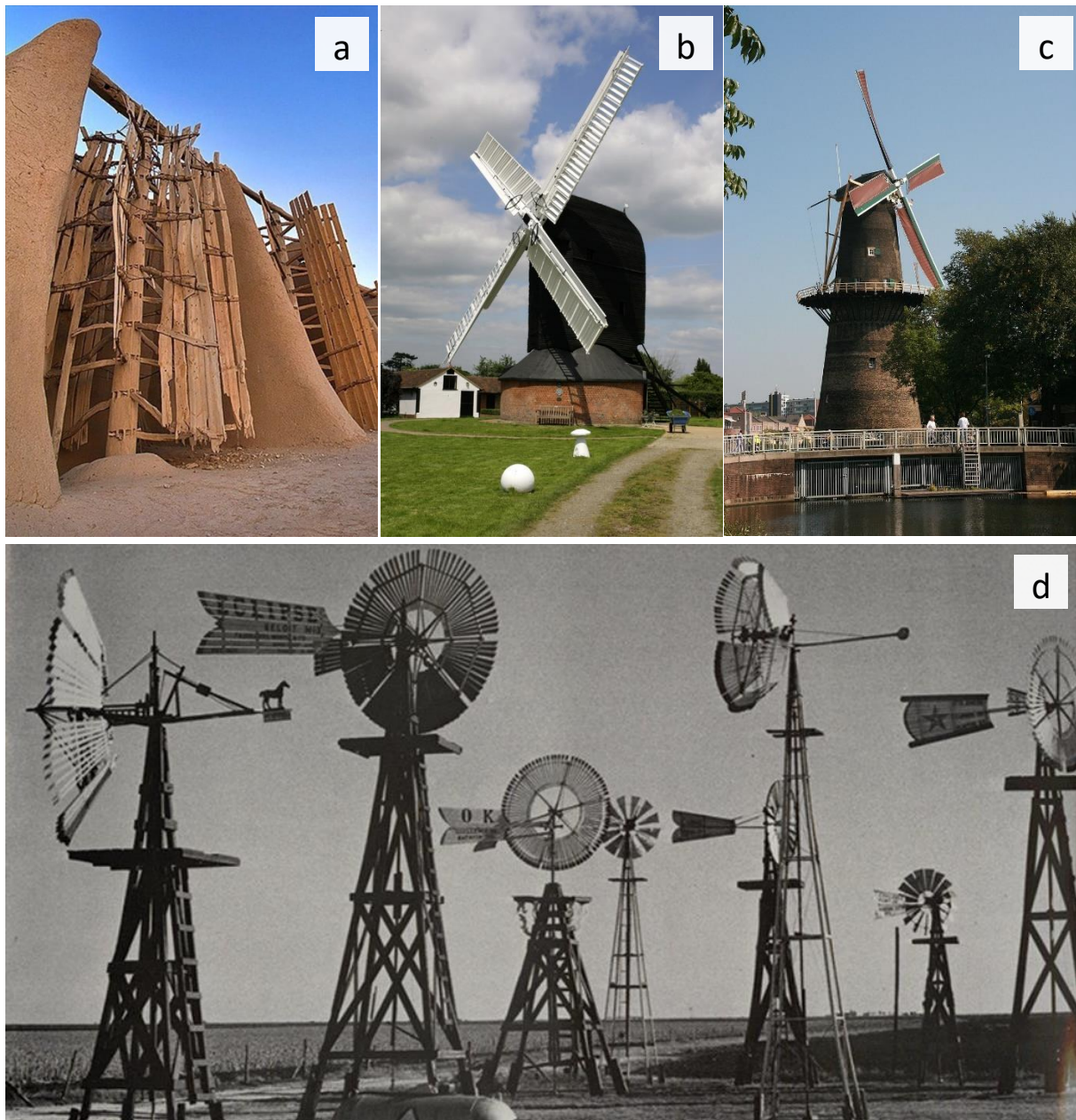
Fig. 1 Evolution of windmills: a) panemone (modern) [14], b) post mill [15], c) tower mill [16], d) American windmill [17]
