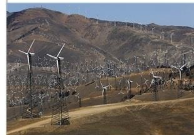
1981: Tehachapi Pass Wind Farm, CA, USA California Wind Rush: first large-scale wind energy penetration outbreak
