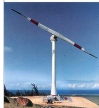
1987: NASA Mod-5B, Oahu, HI, USA The biggest twin-blade HAWT of its times: "power of (big) scale"
