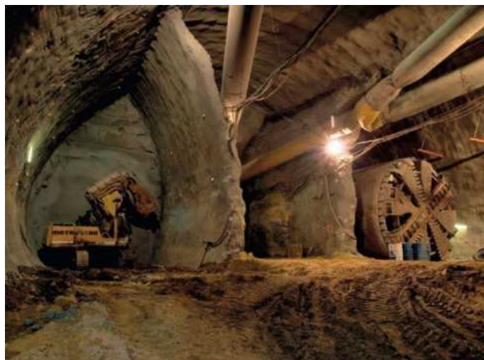
Fig. 1.5 Side drift excavation (Prague subway)
