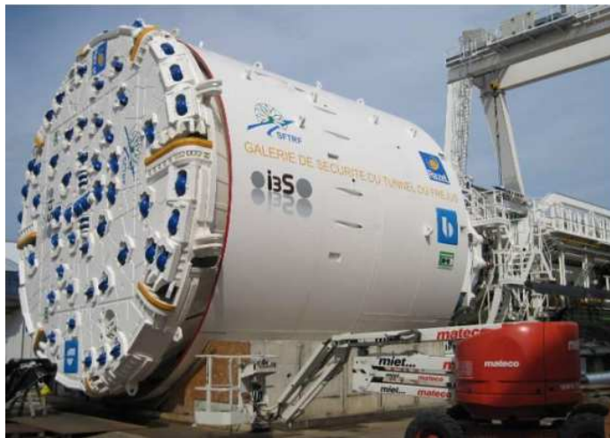
Fig. 6.2 TBM used in the excavation of the safety gallery after Vinnac (2012)
