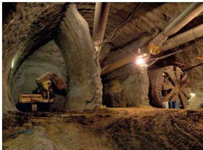
Fig. 1.5 Side drift excavation (Prague subway)
