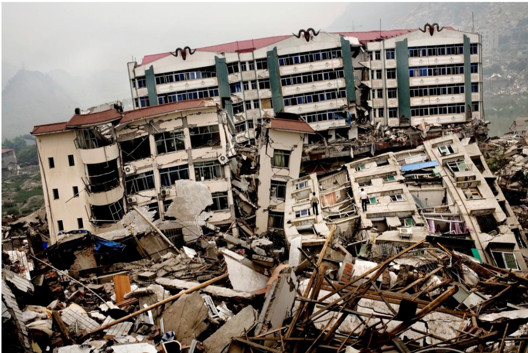
Figure 1.1: Collapsed buildings during the 2008 Wenchuan earthquake ( http://agnesngoy.blogspot.fr )
