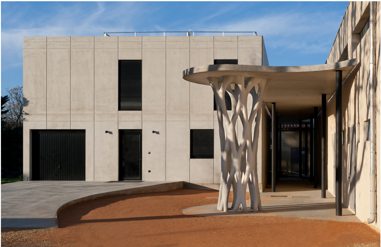
Figure 2.13: Pillar in Aix-en-Provence, XtreeE, 2017
