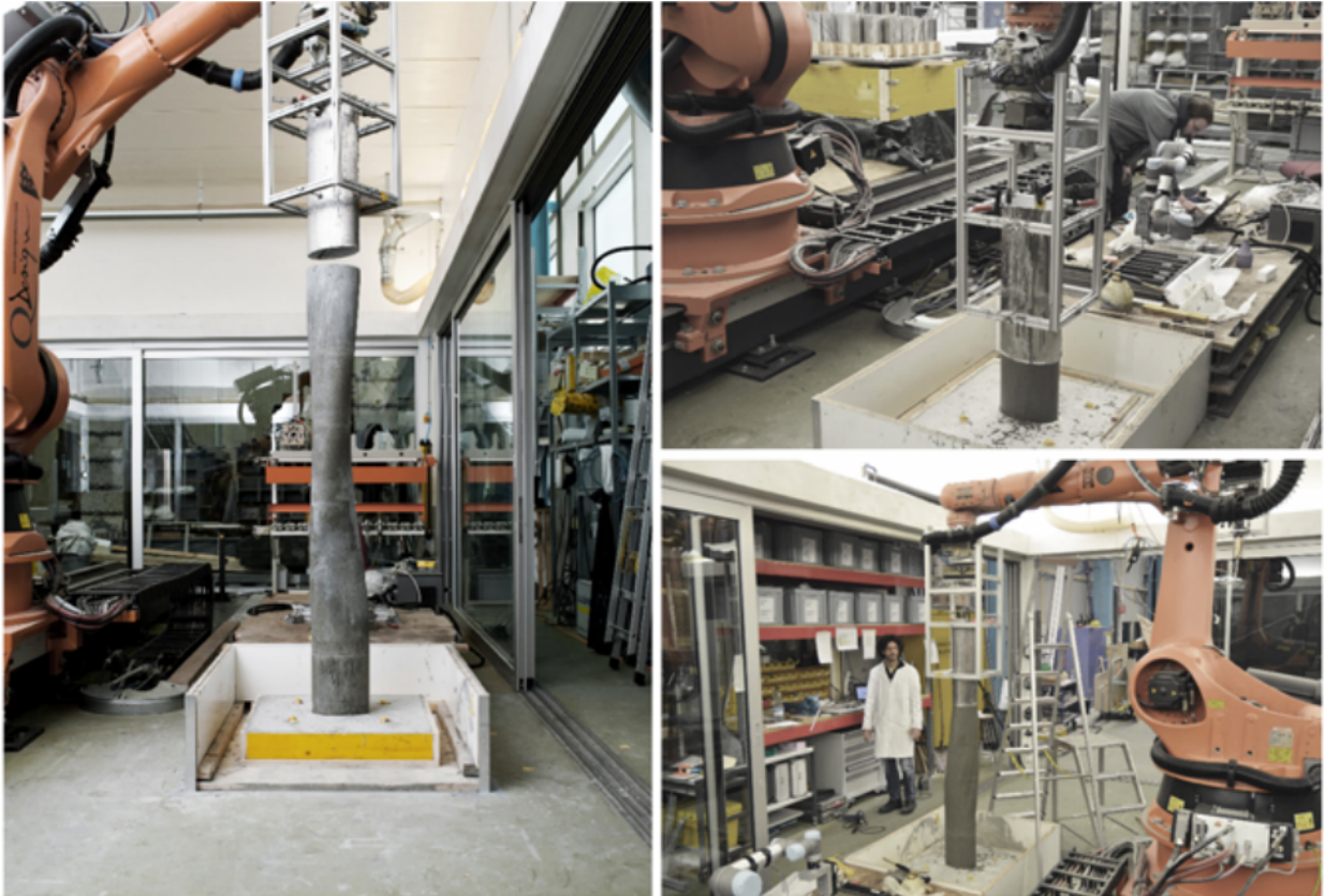
Figure 2.5: Column extrusion by slip forming, published in [50]
