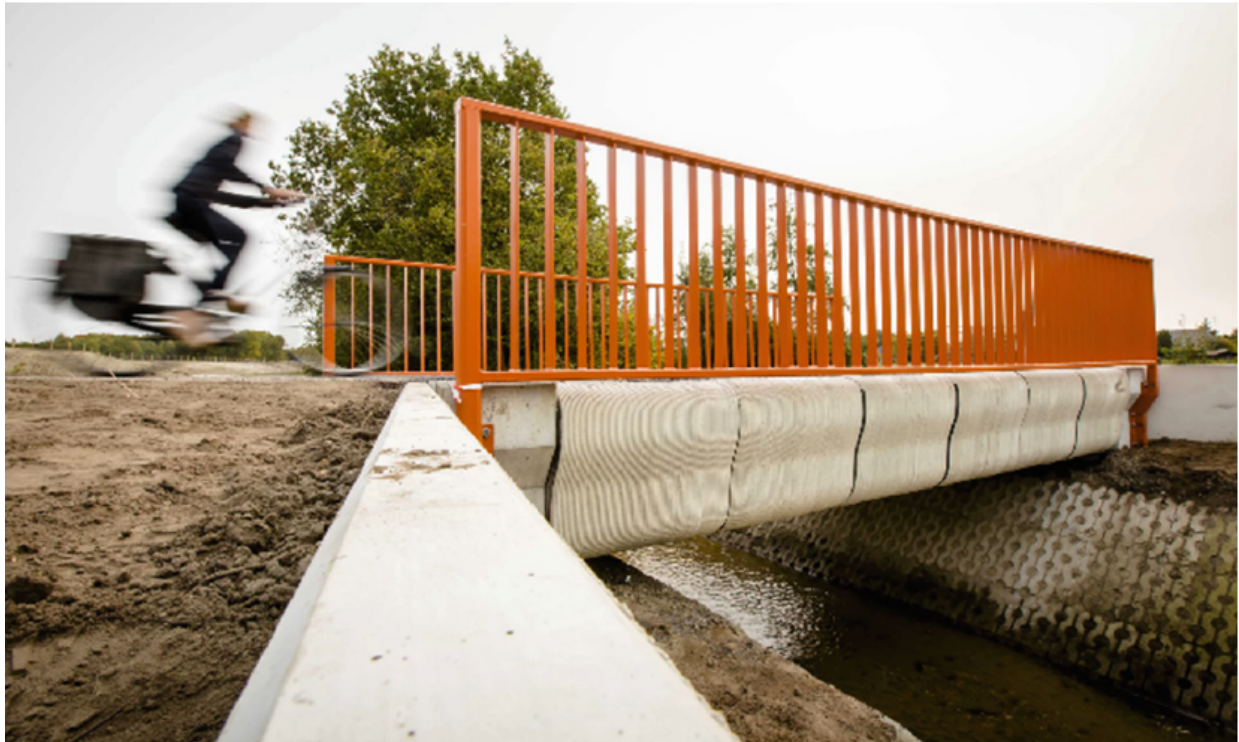
Figure 2.12: TU Eindhoven Bicycle bridge, published in [10]
