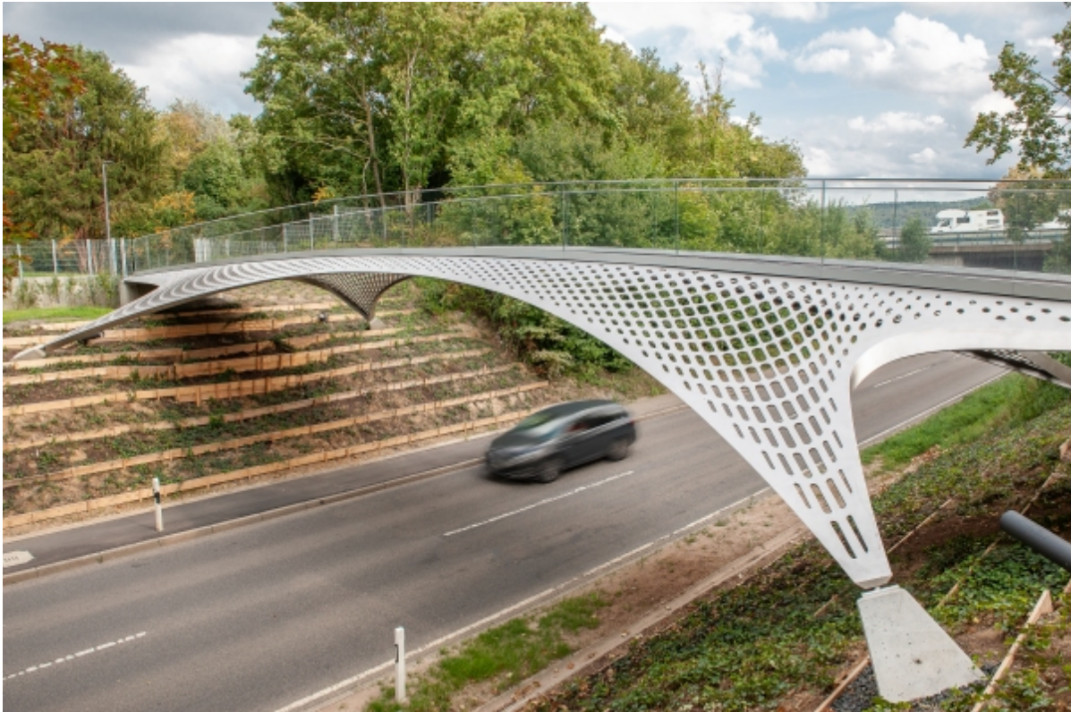
Figure 6.4: Trumpf bridge, Arch. Barkow Leibinger, Ing. Schlaich Bergermann, 2018
