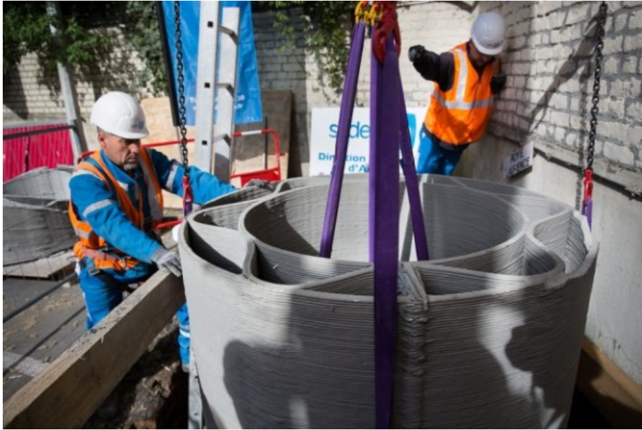
Figure 1.1: Underground inspection pit (XtreeE, 2017). Photography by Anthony Micallef
