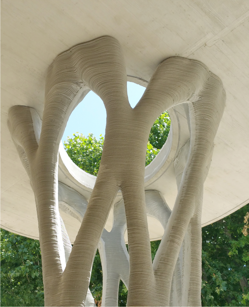
Figure 3.5: Printed pillar in Aix-en-Provence (XtreeE, 2016)
