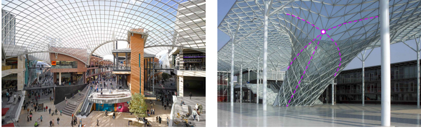
(a) The trimmed quad-mesh pattern of the Cabot Circus Shopping Centre roof in Bristol, England [Schober and Justiz, 2012] (b) The sculpted triangulated quad-mesh pattern of the New Trade Fair in Milan, Italy [Schlaich et al., 2005]
