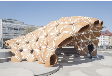
(c) Orientable shape with many handles of the 2015/2016 ICD/ITKE Research Pavilion in Stuttgart, Germany (Source: archdaily.com)
