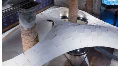
(b) Voussoir tessellation of the Armadillo Vault in Venice, Italy [Rippmann et al., 2016] (Photo credits: Iwan Baan)
