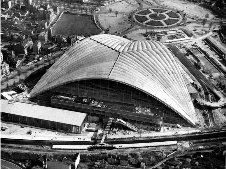
Figure 1.10 – The central singularity of the concrete shell of the CNIT in La Défense, France make the design feasible by orientating the stiffening corrugation pattern towards the supports (source: defense-92.fr).
