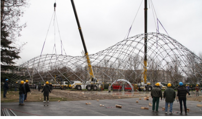
(a) Beam grid of the Ephemeral Cathedral in Créteil, France [Du Peloux et al., 2015] (Photo credits: thinkshell.fr)
