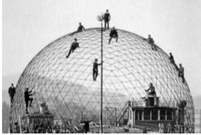
(d) Triangulated pattern of the geodesic dome of the Zeiss-Planetarium in Jena, Germany (Source: zendome.de)
