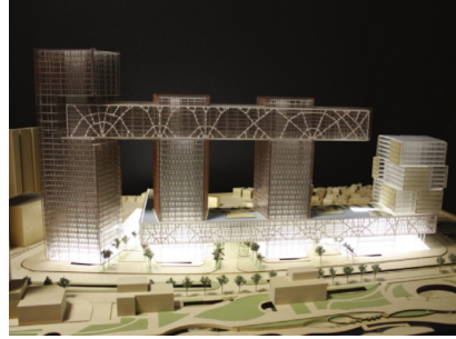
(d) The topology-optimised quad-mesh pattern of the building bridge for the Zendai competition, China [Beghini et al., 2014]
