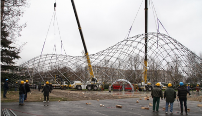
(a) Beam grid of the Ephemeral Cathedral in Créteil, France [Du Peloux et al., 2015] (Photo credits: thinkshell.fr)
