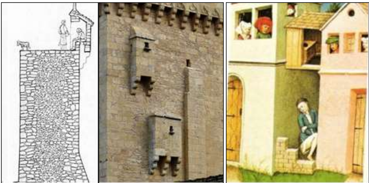
Figure 30 - latrines fixes sans fosse
