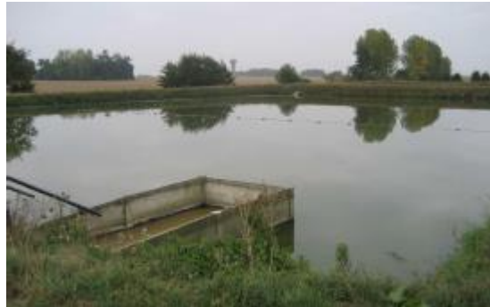
Lagoon system (Chevru, 600 PE)
