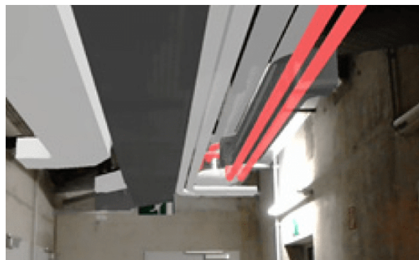
Figure 2.15: Mixed reality application for construction supervision based on superimposition of real and fictive data - Riexinger et al. courtesy [141]
