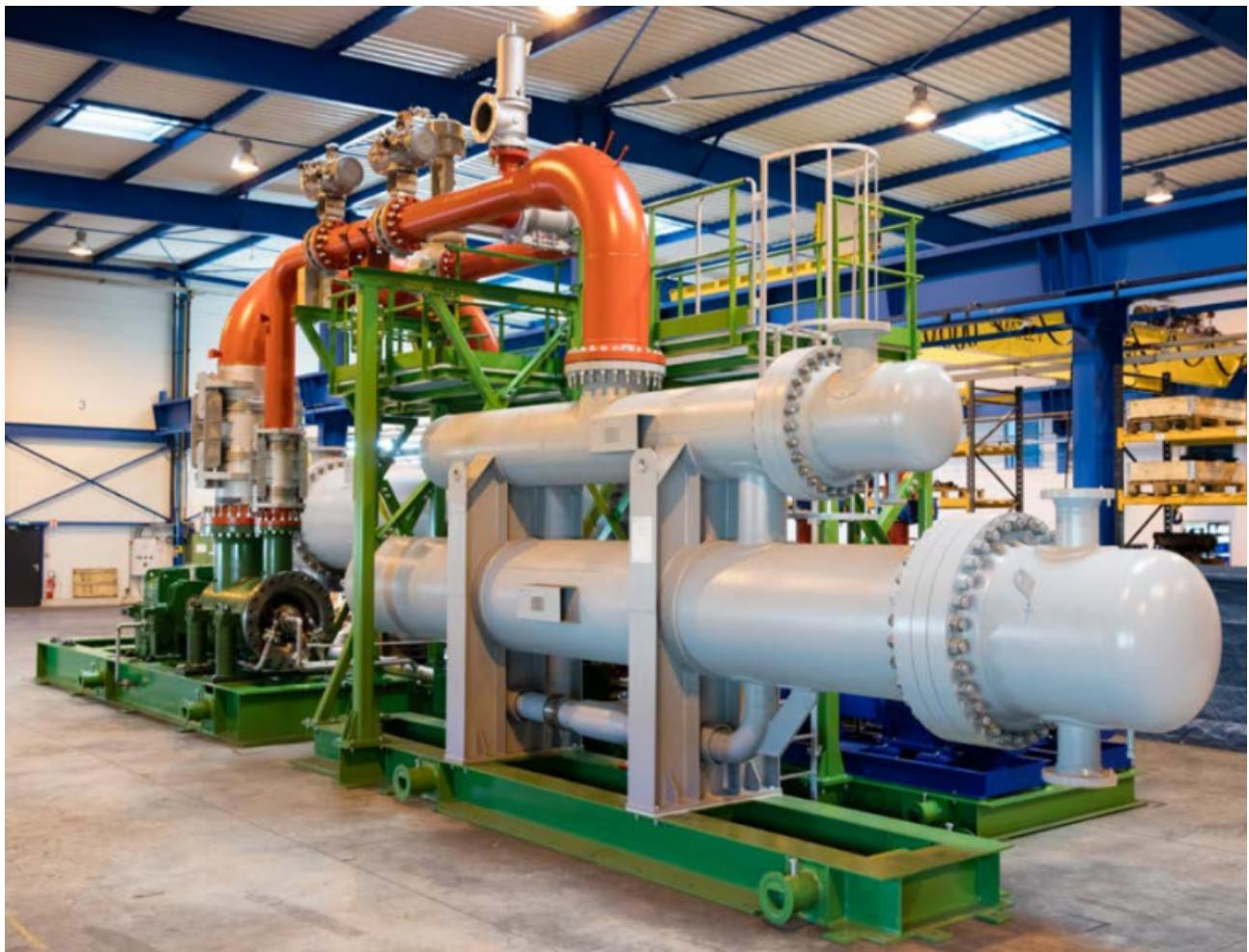
Figure 1.4: Exemple of a 3.2 MW plant for waste heat recovery from a steel mill [3]
