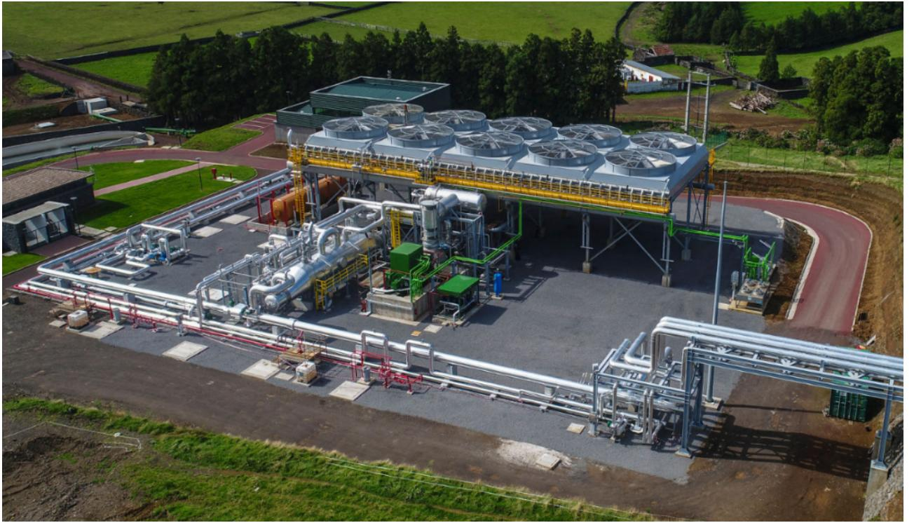
Figure 1.3: Example of application employing a non regenerative one pressure-level cycle [3]
