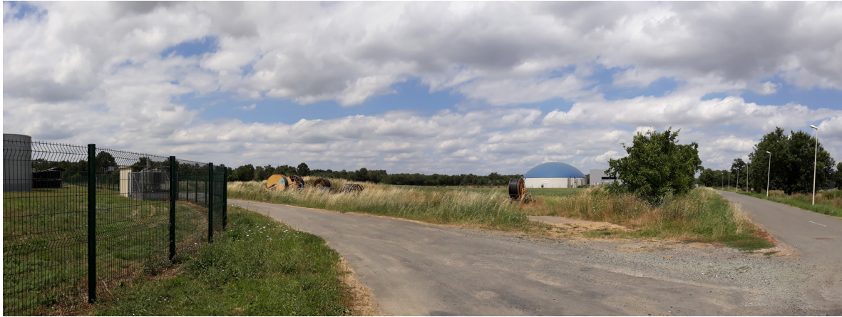
Figure 3. Cap'Ter biogas power plant in Saint-Varent's industrial area, CC Thouarsais. Source: author July 2018
