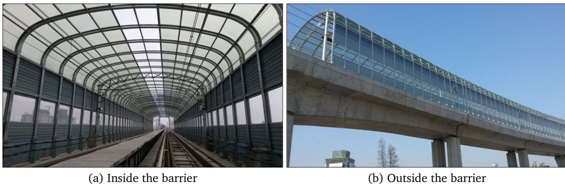
Fig 1.2.: A prototype of a nearly-enclosed barrier located in Ningbo, China
