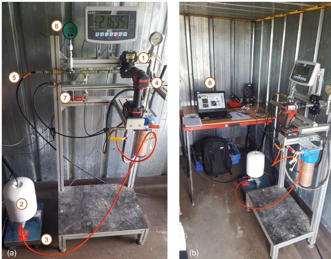
Figure 3.2 – (a) Photo of the pressure-volume controller (principle patented by Cour (2017)) ; (b) view of the setup on site showing data acquisition;
