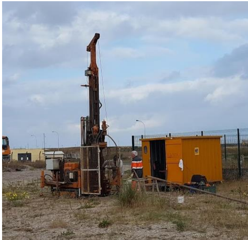
Figure 3.5 – General view of the testing setup at Dunkirk site
