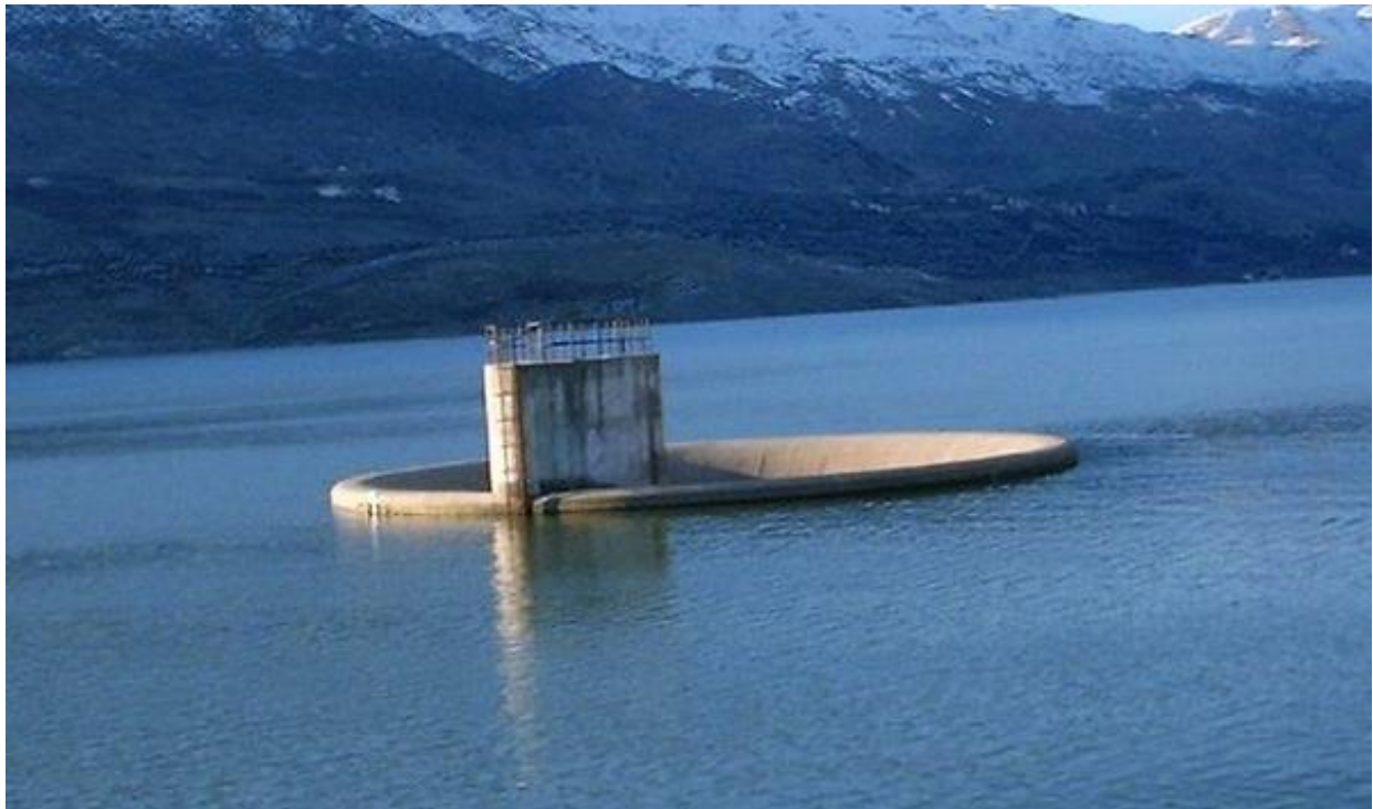
Figure 8: Spillway at Karaoun Reservoir, Lebanon ( www.litani.gov.lb ).
