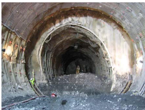
(a) Large and anisotropic cross-section closure
