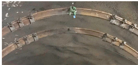
Figure 1.13: TH type steel ribs with sliding joints
