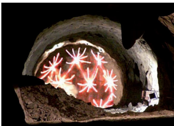
(a) Drill and blast excavation
