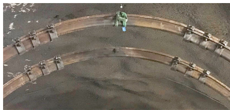
Figure 1.13: TH type steel ribs with sliding joints
