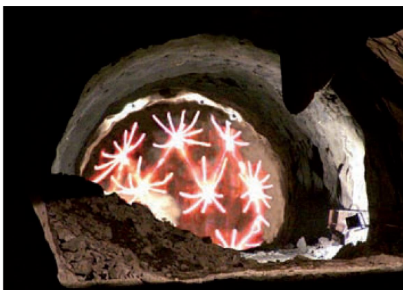
(a) Drill and blast excavation
