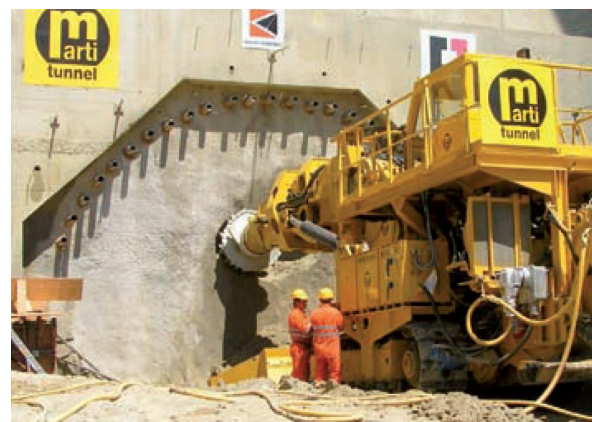
(b) Roadheader excavation
