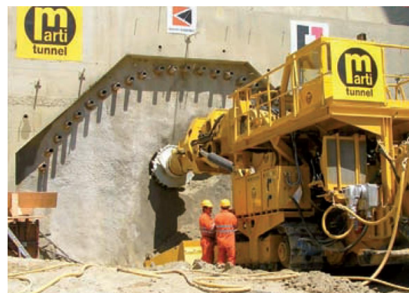
(b) Roadheader excavation
