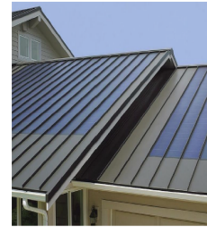
(c) Roof made with sandwich material
