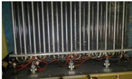
Figure 3.13: Herringbone fin-and-tube heat exchanger (CFX).
