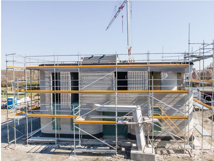
Figure 1.2: 3D printing of a house by (Peri [2020]).
