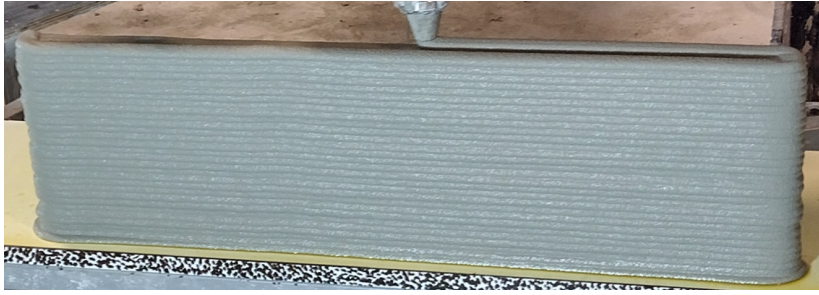
Figure 1.1: Printing a wall by layer-wise concrete extrusion.
