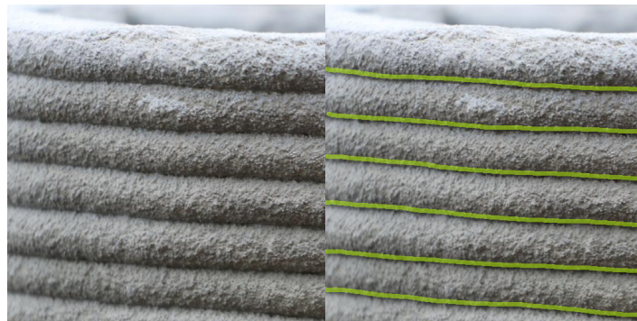
Figure 4.1: Example of interlayer lines on a dry piece produced by 3DCP. The interlayer lines are highlighted in green.
