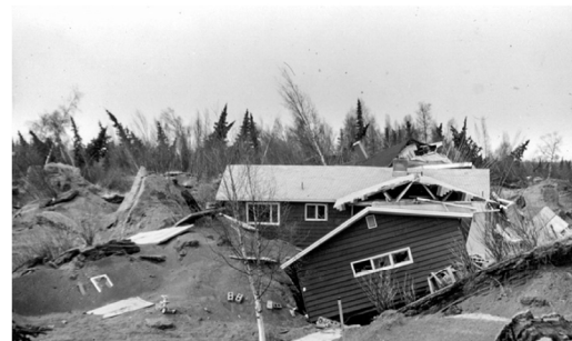
Figure 1.1 Photographic views of liquefaction disasters: (a) Niigata earthquake; (b) Alaska earthquake (Niigata earthquake from https://en.wikipedia.org/wiki/Soil_liquefaction and Alaska earthquake from https://en.wikipedia.org/wiki/1964_Alaska_earthquake ).
