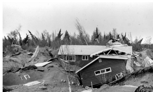
Figure 1.1 Photographic views of liquefaction disasters: (a) Niigata earthquake; (b) Alaska earthquake (Niigata earthquake from https://en.wikipedia.org/wiki/Soil_liquefaction and Alaska earthquake from https://en.wikipedia.org/wiki/1964_Alaska_earthquake ).
