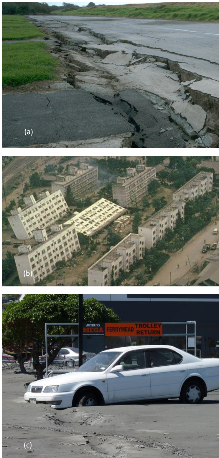
Figure 1-1 – Damage caused by soils liquefaction during earthquakes, (a) Loma Prieta 1989 (USGS 1989) , (b) Niigata 1964 (Ishihara and Koga 1981) and (c) Christchurch 2011 (GEONET 2022).
