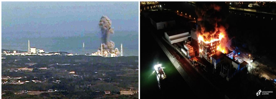
Figure 1.2: Consequences of a bad design, monitoring or exploitation of industrial buildings. (Left) Fukushima accident in 2011 caused by an hydrogen explosion after the endomagement of the primary cooling cycle by an earthquake (credits: Fukushima Central Television). (Right) Fire at a data centre in Strasbourg in 2021 (credits: Sapeurs Pompiers du Bas Rhin), due to an overheat of two inverters. Moreover, given the building design, the firefighter could not have a proper access to the burning devices. Additionally, the centre architecture (which used a free cooling ventilation strategy) accelerated the fire dispersion (Lawrance, 2020).
