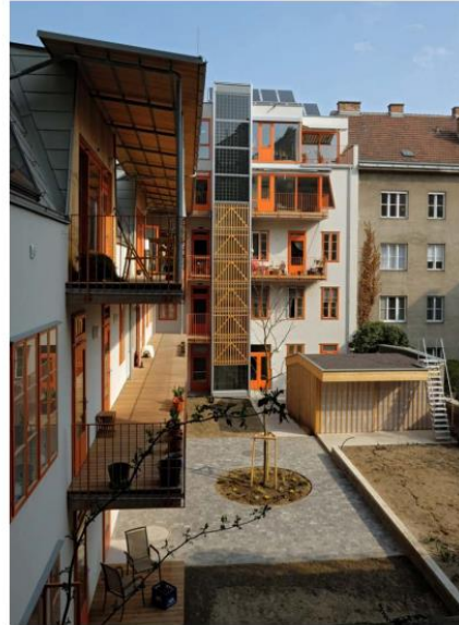
Inner yard after accomplishment of drillings, Source: © Lisi Zeininger
