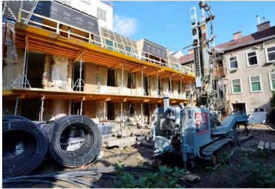
Operating drilling rigs in the inner yard of the building, source: ÖGUT
