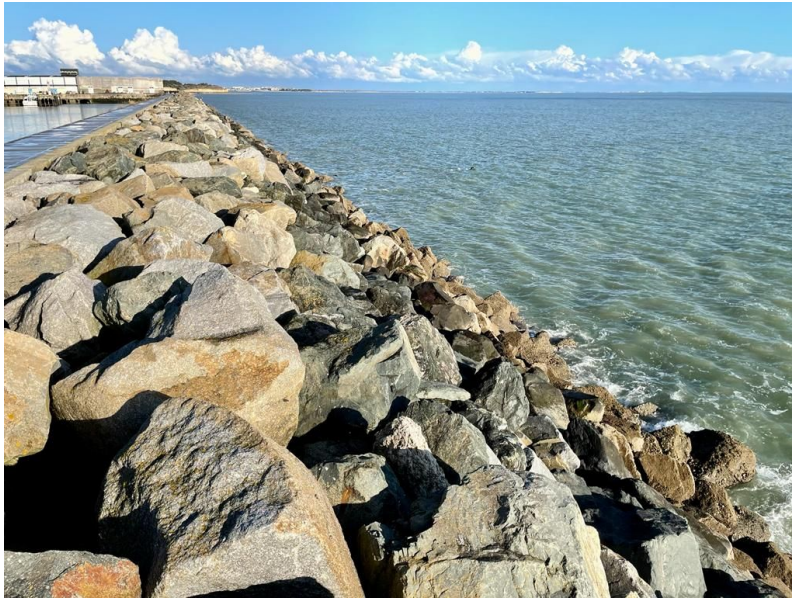
Figure 5.2: Photograph of an armoured rubble-mound breakwater (in La Pallice harbour, La Rochelle, France) similar to the model considered in the present study (photo: Hubert Branger).
