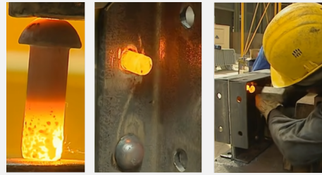
Figure 2.1 | A rivet is heated, and inserted in the parts before its end is hammered. Renovations of the Grand Palais, Paris, France. Source: [1].
