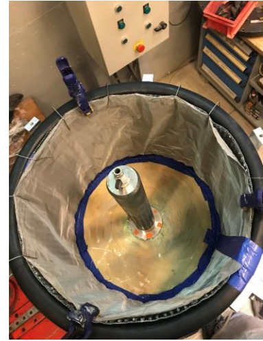
c – installation of the lateral drainage system
