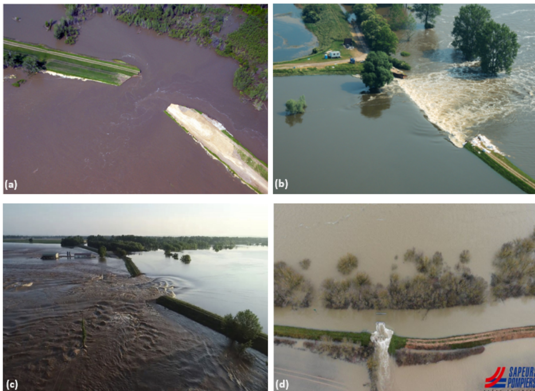
Figure 4: Examples of levee failure cases: (a) Levee breach near Hamburg in 2011 ( www.floodfactor.com ), (b) Levee failure on the Elbe river in 2013 (Jüpner (2015)), (c) Levee breach along the Arkansas river in 2019 ( www.detroitnews.com ), (d) Levee failure along the Saône-et-Loire in 2021 ( www.lejssl.com ).
