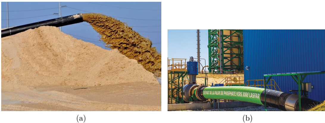
Figure 1.1: OCP phosphate slurry pipeline. Crédit photo : OCP, 21/01/2021
