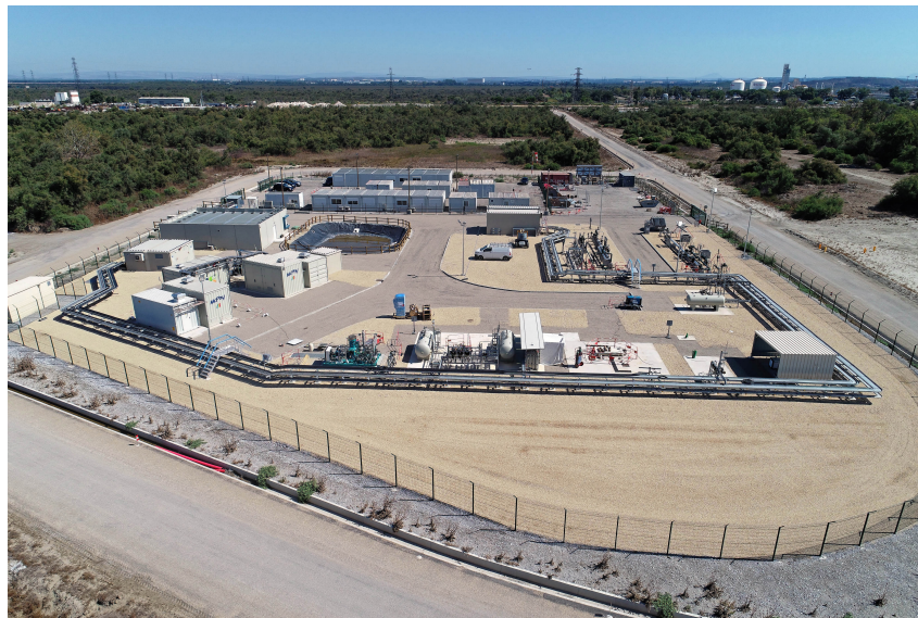
Figure 1.28: The Jupiter1000 Power-to-Gas plant in Fos-sur-Mer, France, reprinted from [109].
