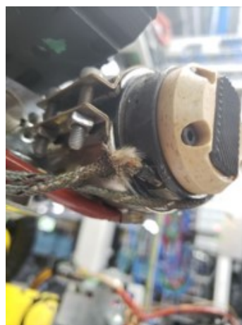
Figure E.2: Thermocouple cable issue
