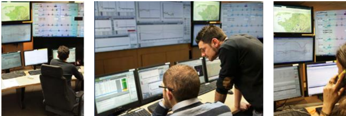
Figure 2: the central control room managing flow via the 440 km sewer network towards the wastewater treatment plants and storm water retention basins. (© SIAAP)
