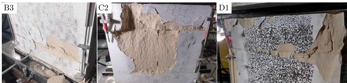
FIGURE 8.25 – Rupture en compression/délaminage de la pierre
