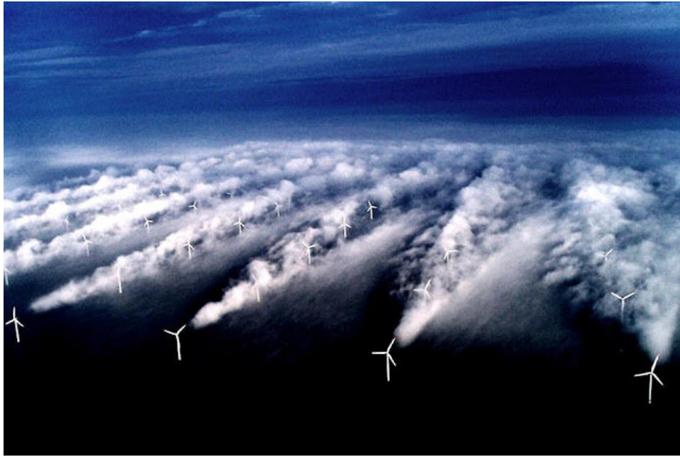
Figure 2.4: Offshore wind farm Horns Rev 1 in Denmark. Photograph by Christian Steiness / Vattenfall.
